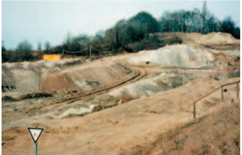
Figure 11 Road works construction site
